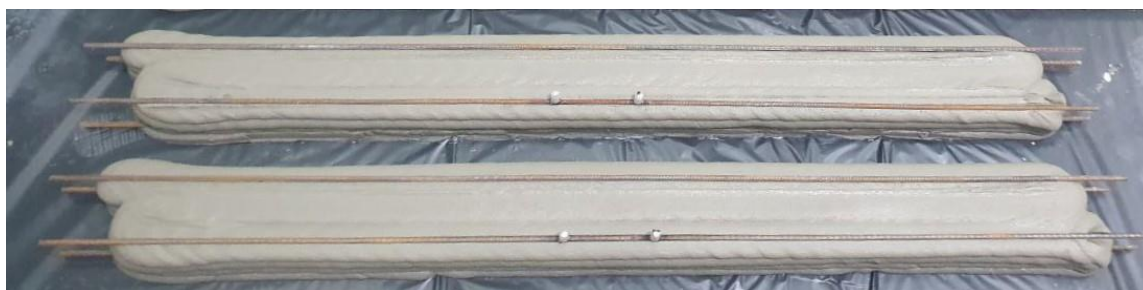
Fig. 5. Placement of individual reinforcing bars on the fourth layer
